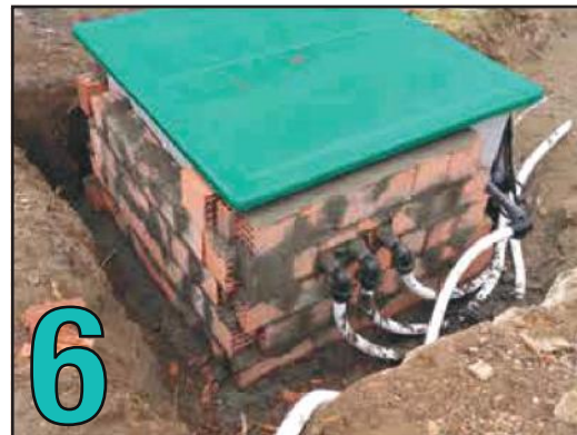
Preparation and protection of machine room.
