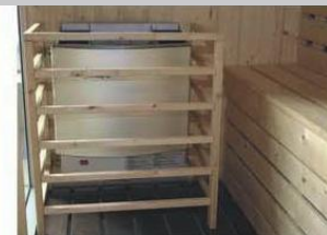
Wooden frame for protecting sauna heat generator
